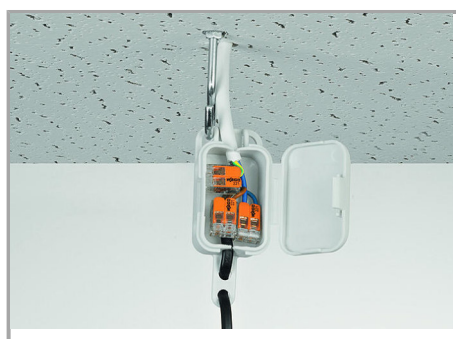
Pendant light connection in suspended ceilings
