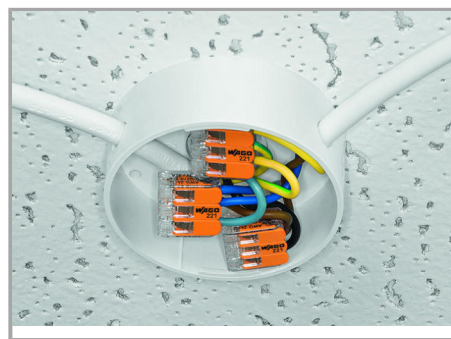
Lighting distribution in ceiling canopy
